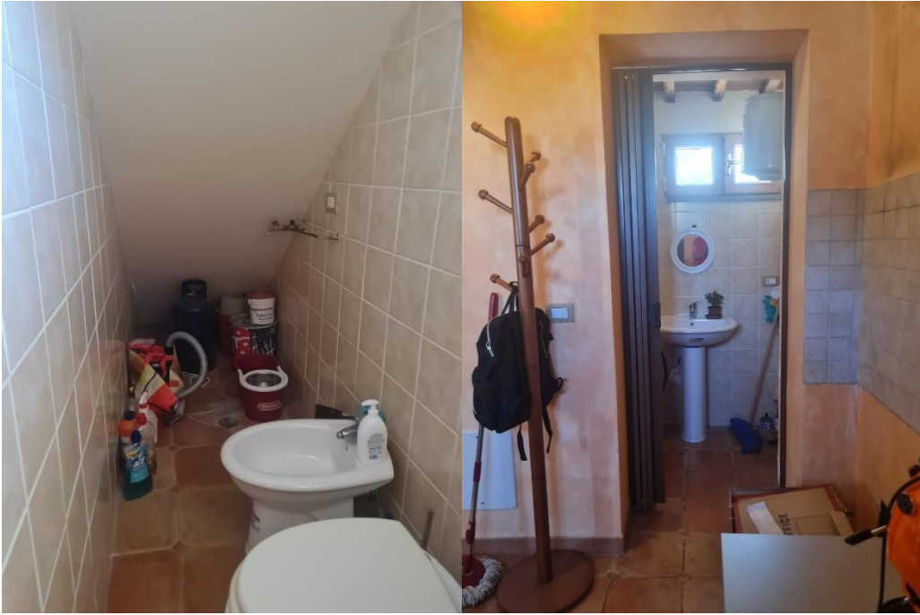
Bagno piano terra
