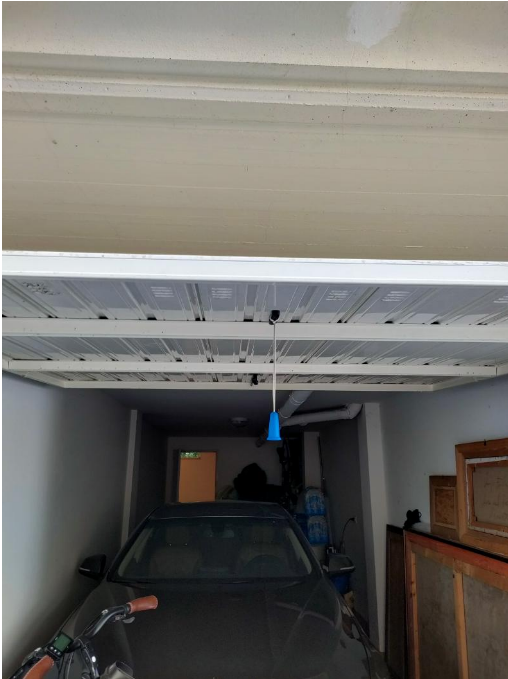
Vista Garage al Piano Seminterrato
