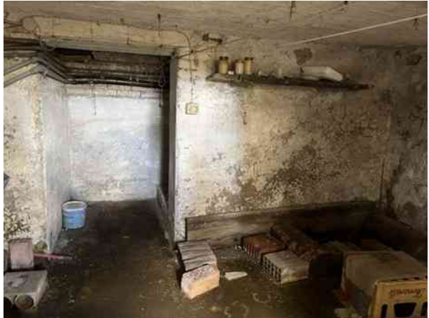
Cantina – piano interrato
