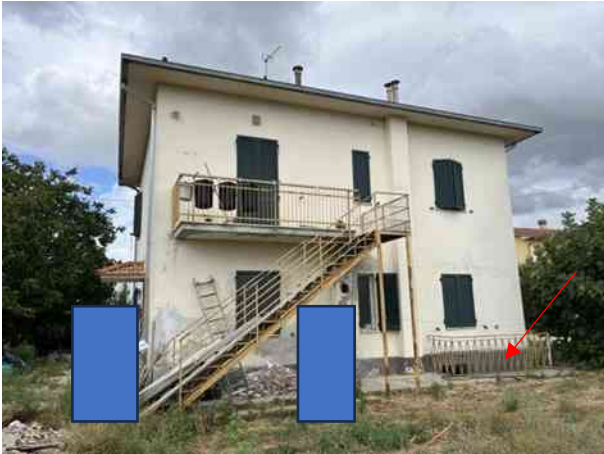
Cantina – piano interrato
