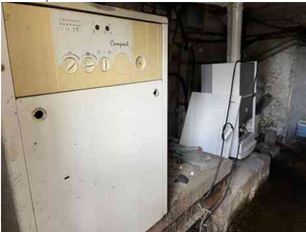
Cantina – piano interrato
