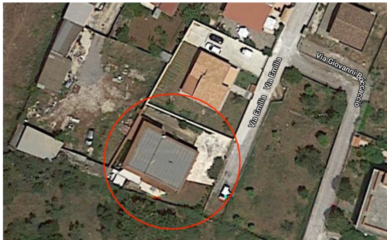
(Foto aerea Google Maps 09/02/2021);
