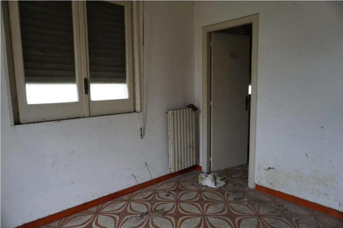
Fig.23 – Vista vano interno dell’immobile sub.9 (A10)
