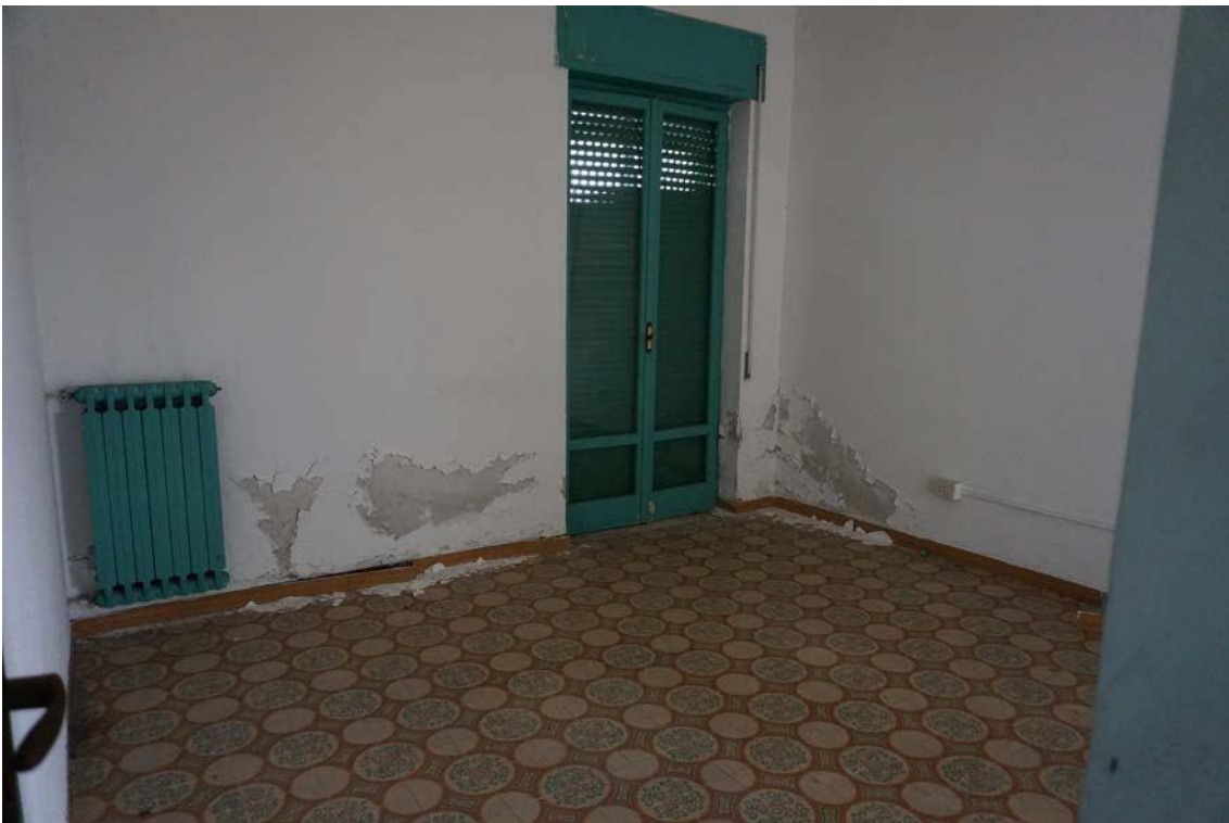
Fig.74 – Vista vano dell’immobile sub.13 (A10)
