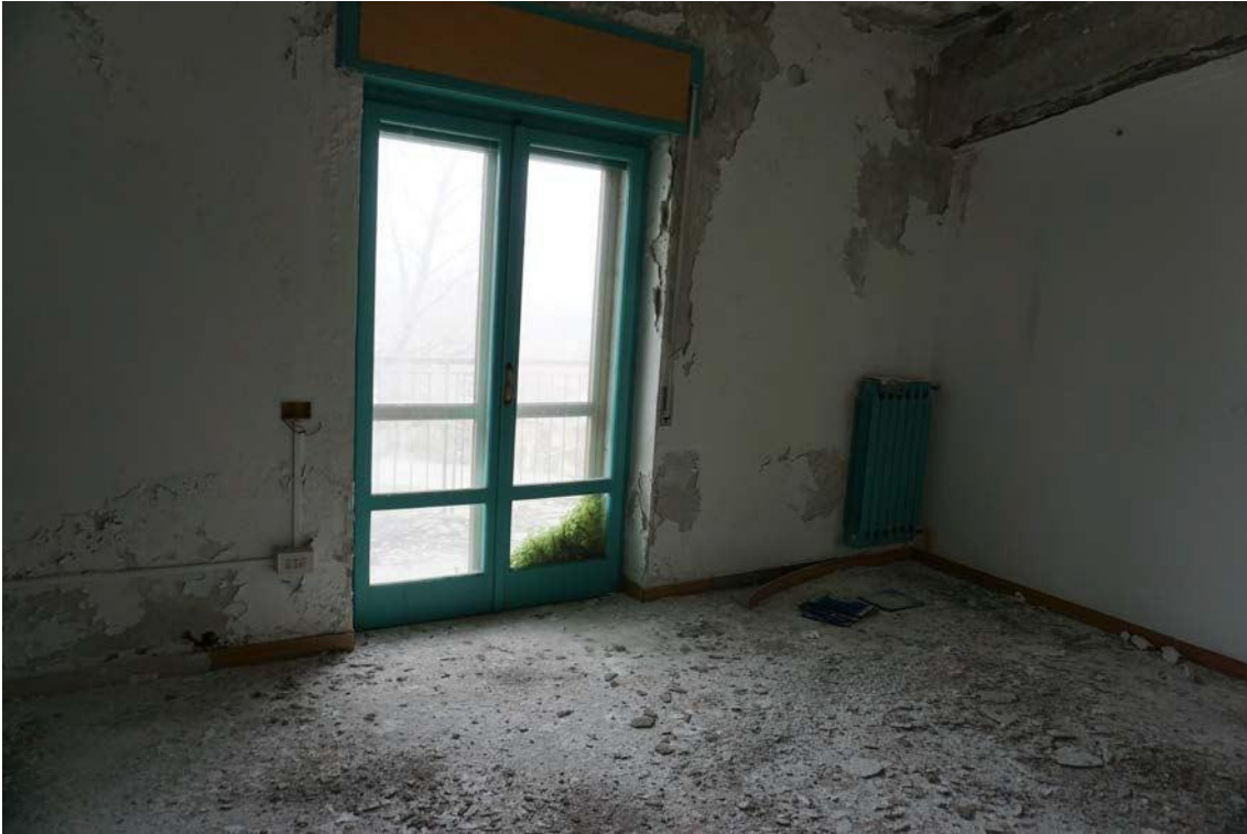
Fig.75 – Vista vano dell’immobile sub.13 (A10)
