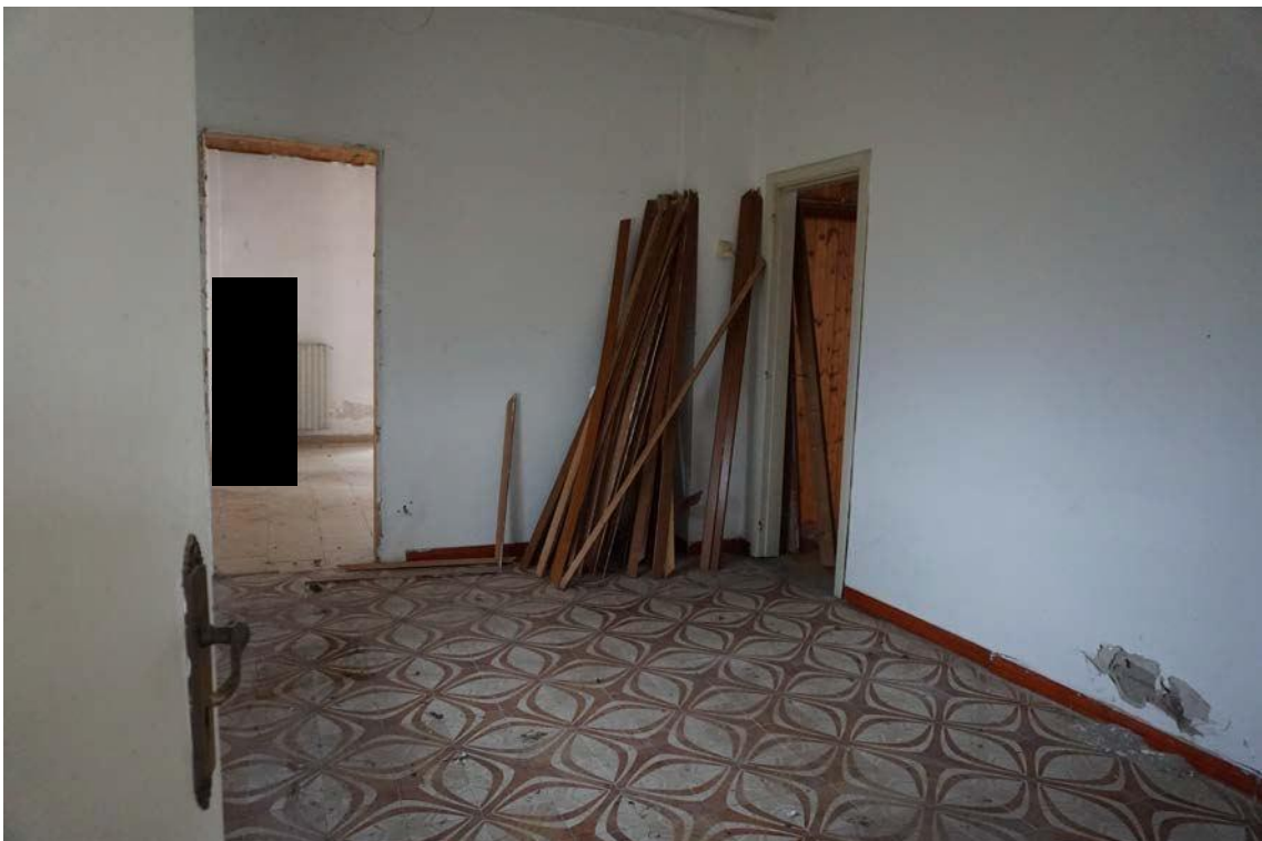
Fig.24 – Vista vano interno dell’immobile sub.9 (A10)
