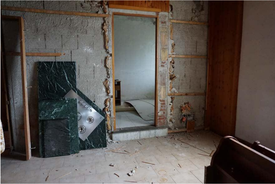
Fig.25 – Vista vano interno dell’immobile sub.9 (A10)
