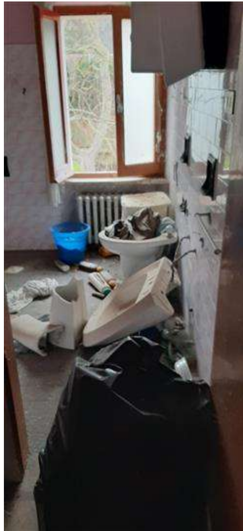
Bagno Piano Terra
