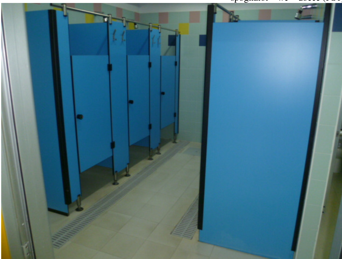
spogliatoi – wc – docce (PS1)
