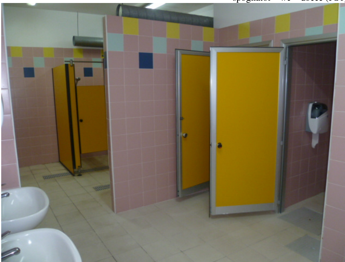
spogliatoi – wc – docce (PS1)
