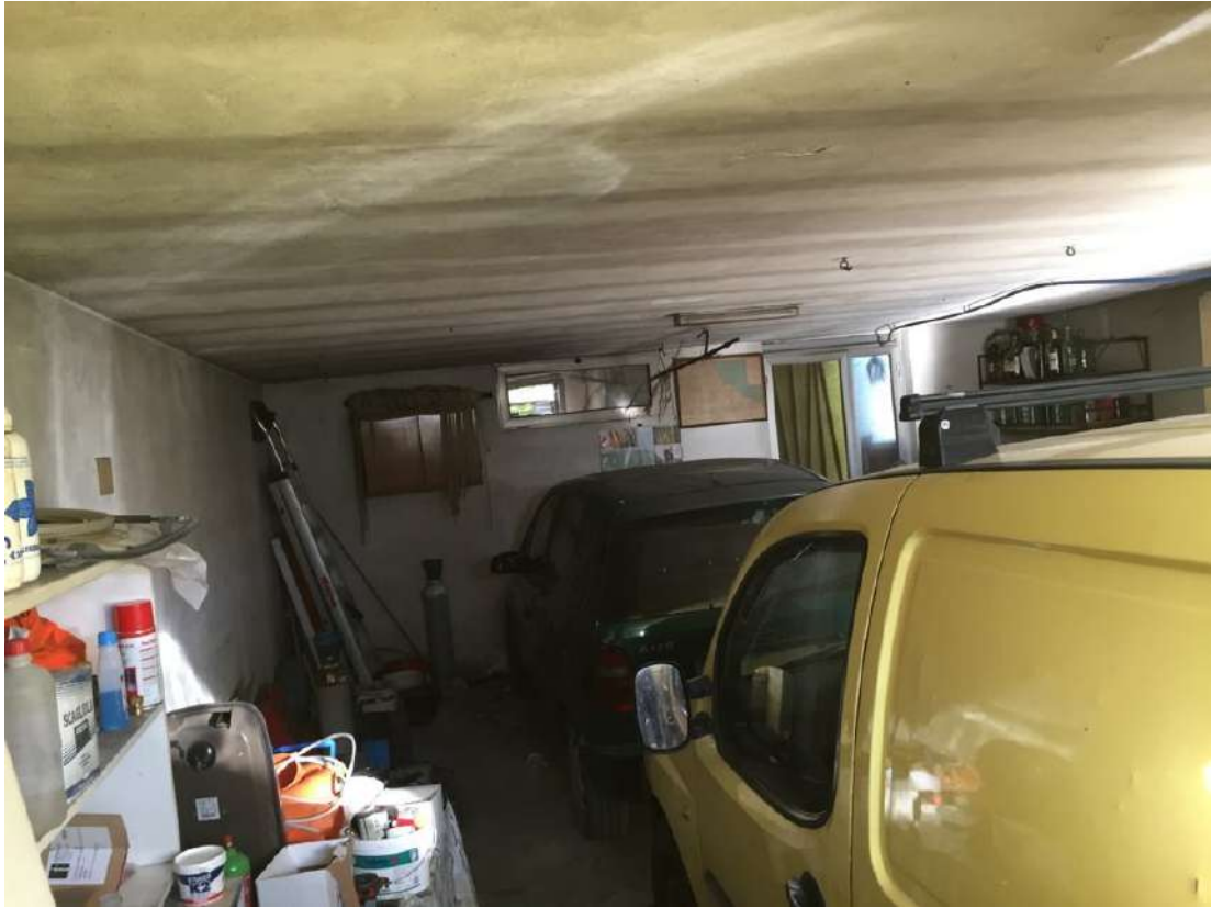
Foto 11 – Garage Piano Terra
