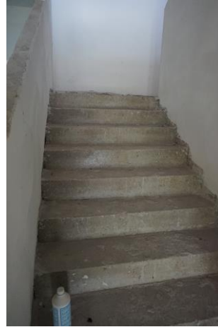
Piano terra – Scala interna
