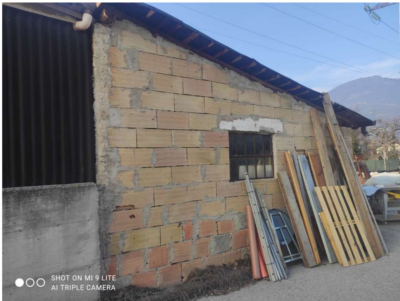
Figura 11: C.C. VILLALAGARINA P.ED. 410 (facciata est).
