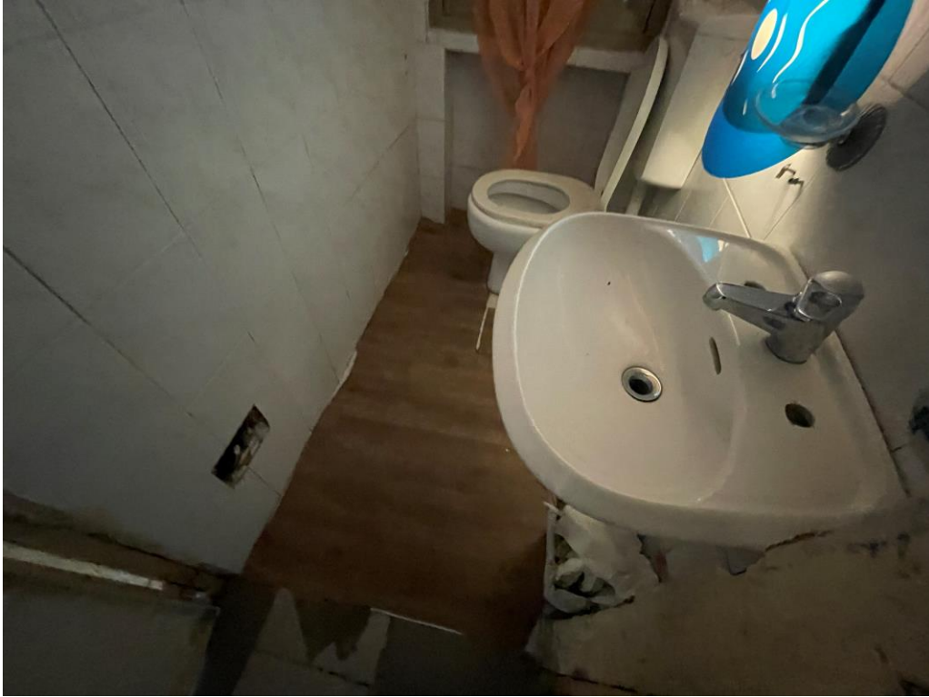
Bagno piano terra
