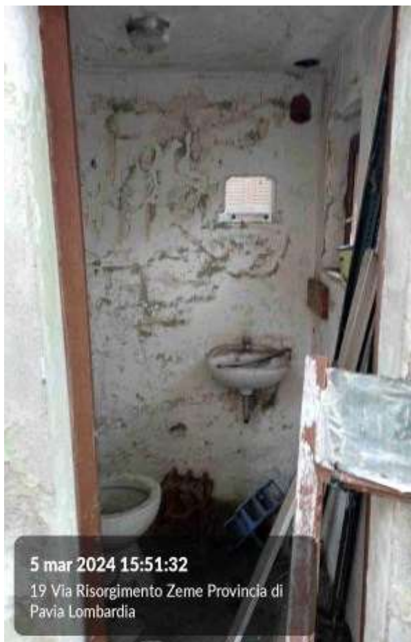
Locale bagno in cortile
