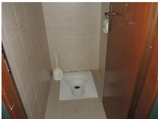
WC a piano terra
