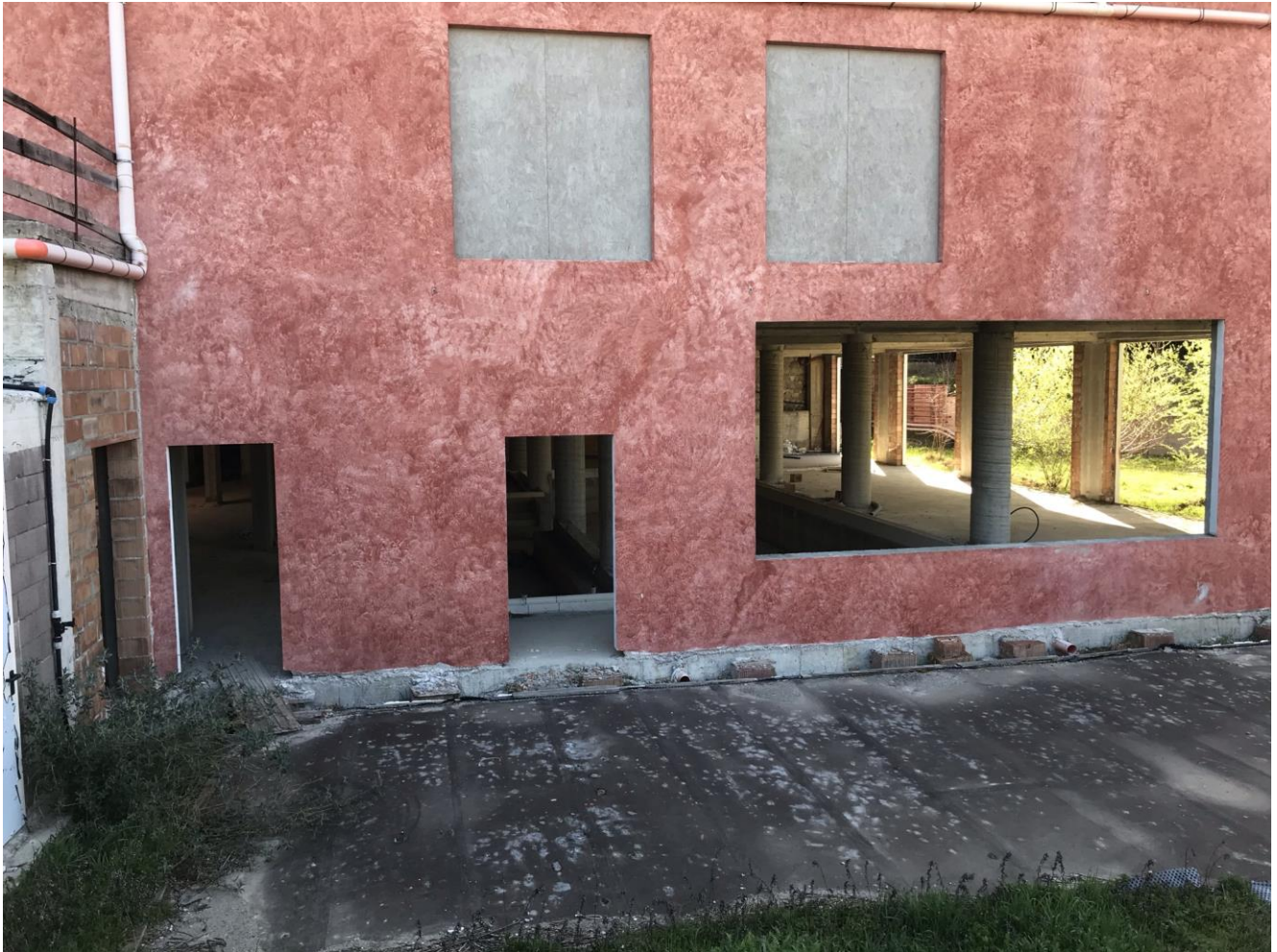
Scorcio piano interrato
