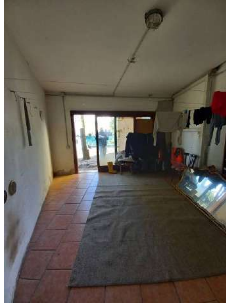
VISTA GARAGE SUB 10
