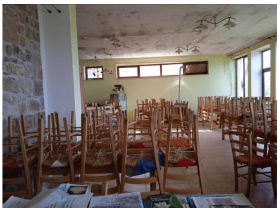
Part. 477 - Vista interna piano terra
