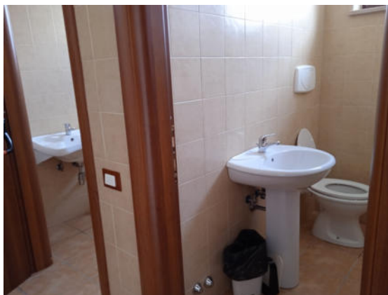
Part. 477 - Vista interna piano terra
