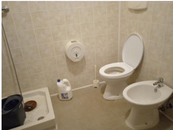
Part. 476 sub 2 - Vista interna piano terra
