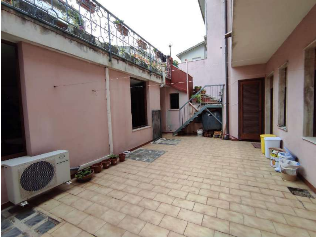
Figura 31- vista 27, sub.5, terrazza
