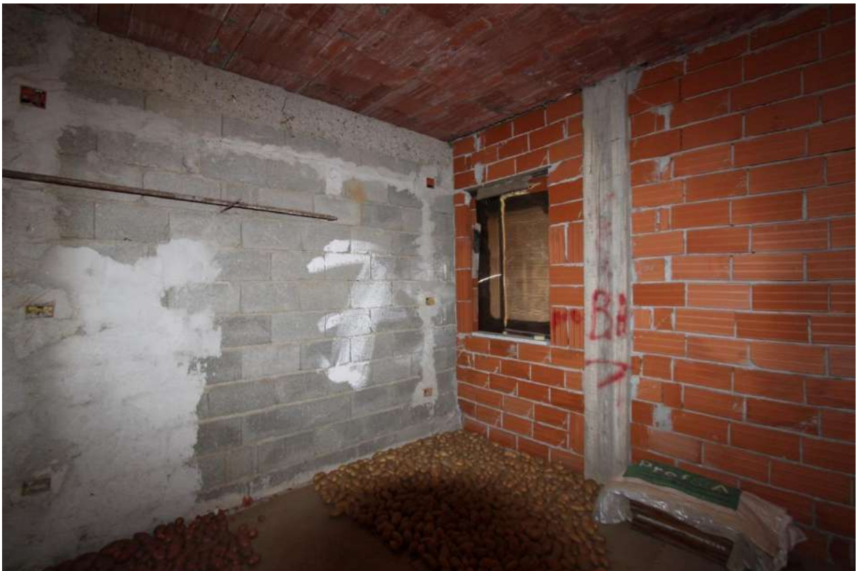
Figura 61- vista 58, camera piano terra
