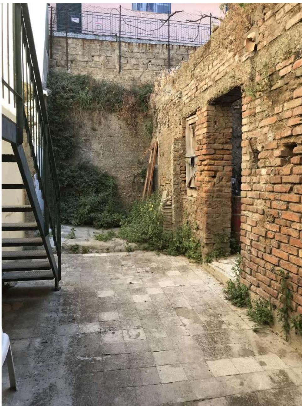
Cortile piano terra
