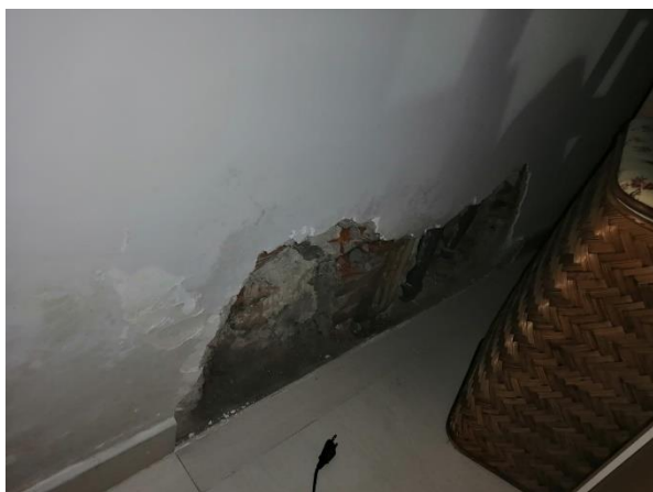
Vista Interna camera L2
