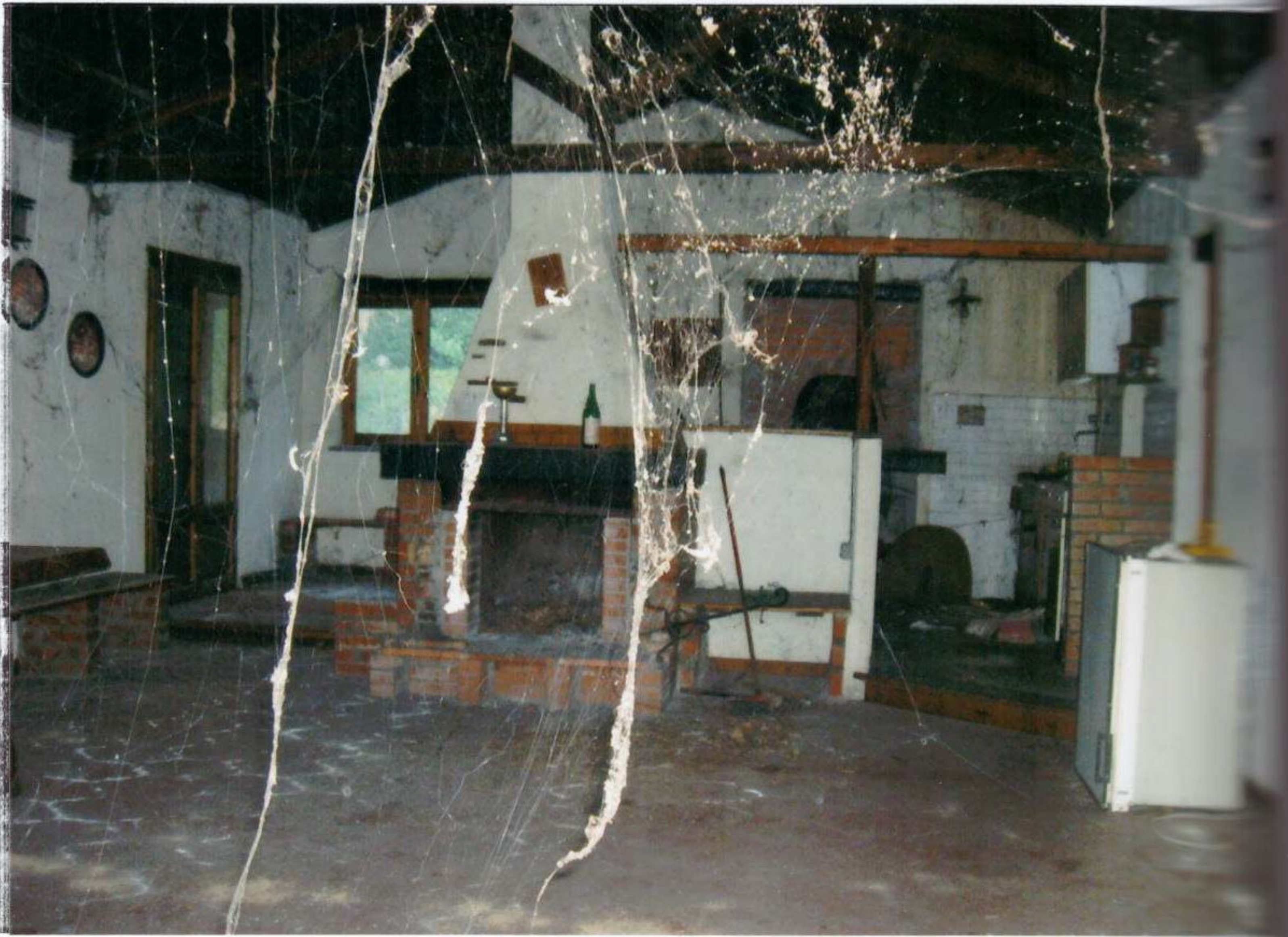
VISTA INTERNA ALTA DEBANDANCE
