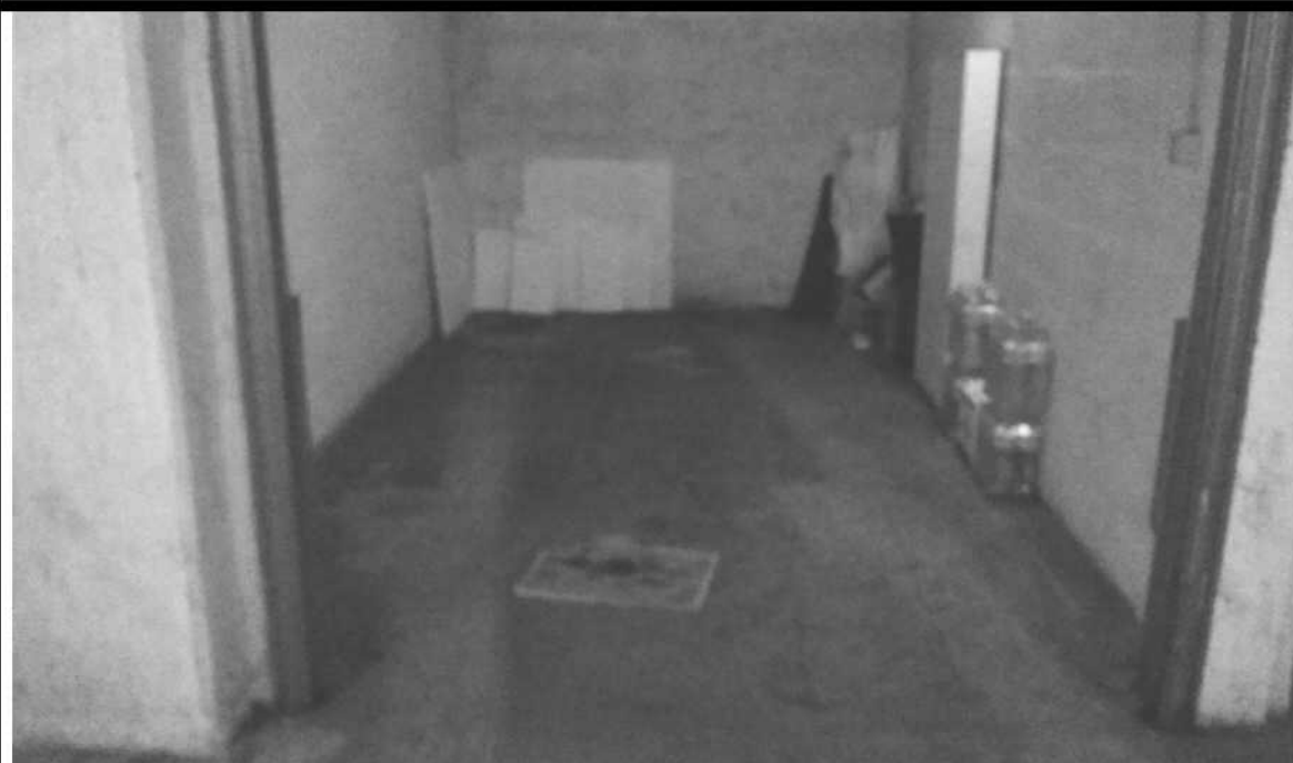
FOTO 144 – VISTA AUTORIMESSA – BOX 19 – PIANO SEMINT.
