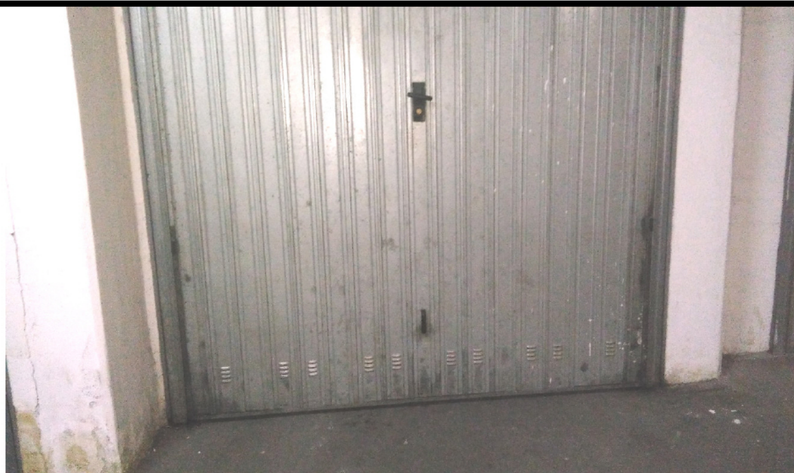
FOTO 141 – VISTA AUTORIMESSA – BOX 18 – PIANO SEMINT.
