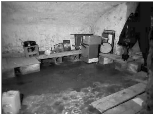
13. Cantina piano interrato
