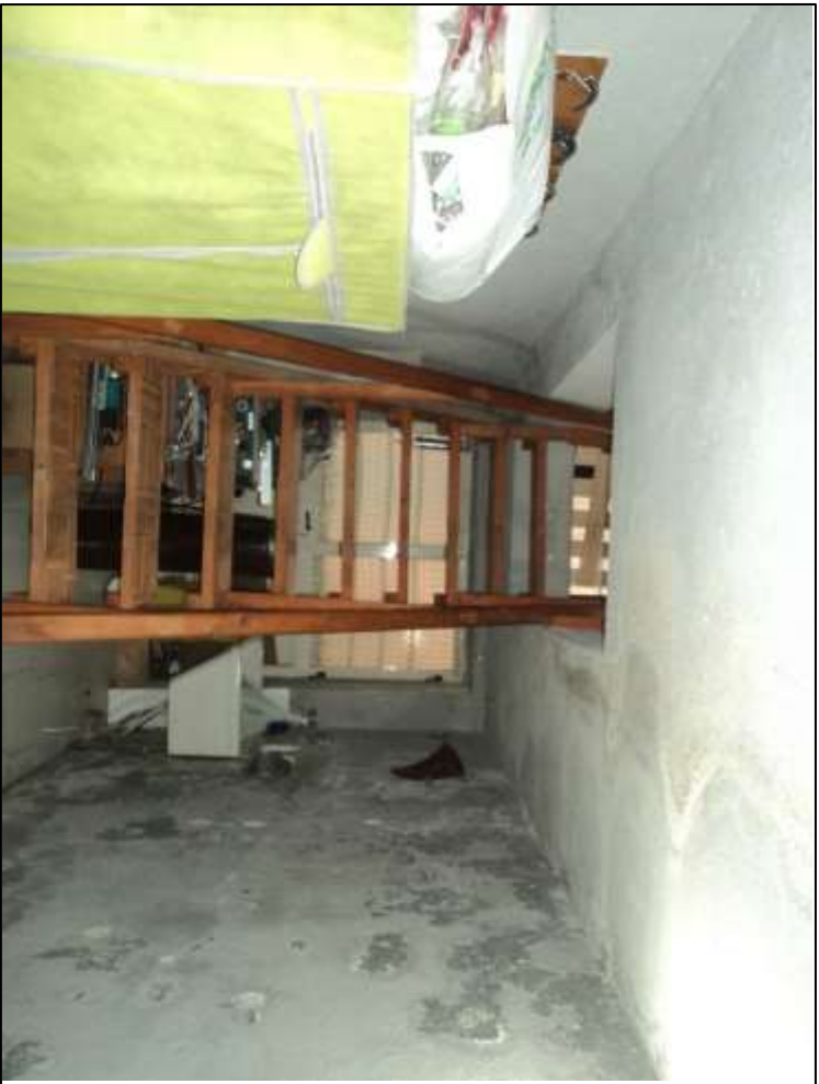
Piano seminterrato – botola scala
