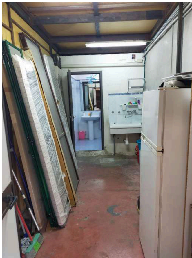
Interno (locale wc)
