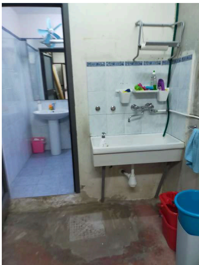
Interno (locale wc)
