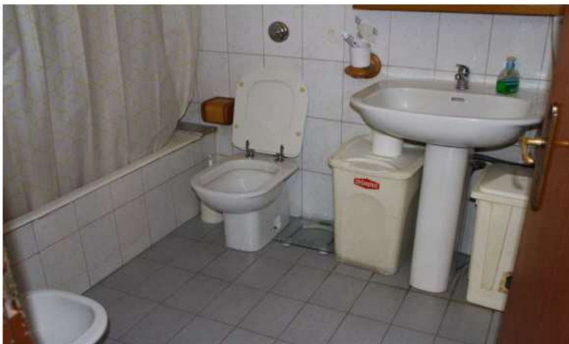
Bagno Piano Terra
