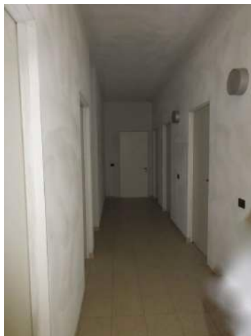
cantine piano interrato
