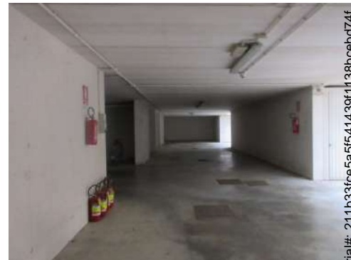
Piano interrato - garage
