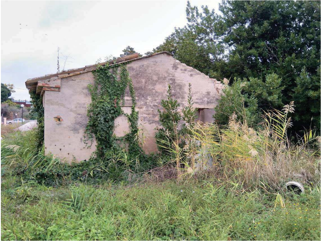
Foto 25. Locale garage – piano terra
