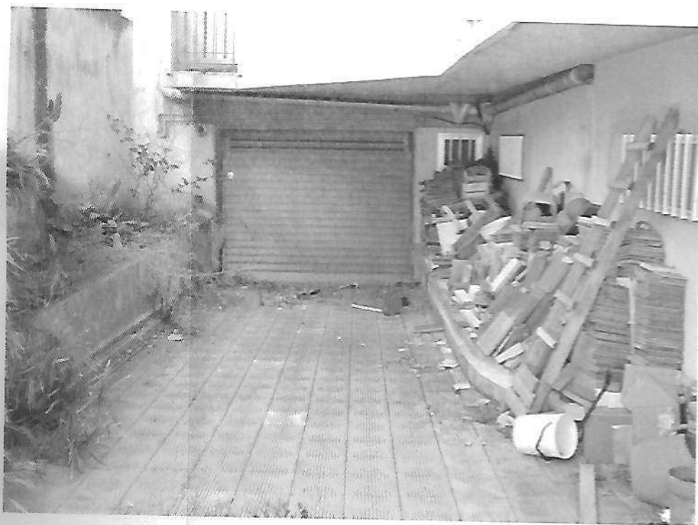
Foto 03 – locale garage – sub 2
