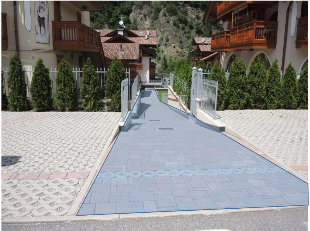
Rampa p.ed. 563 p.m. 37
