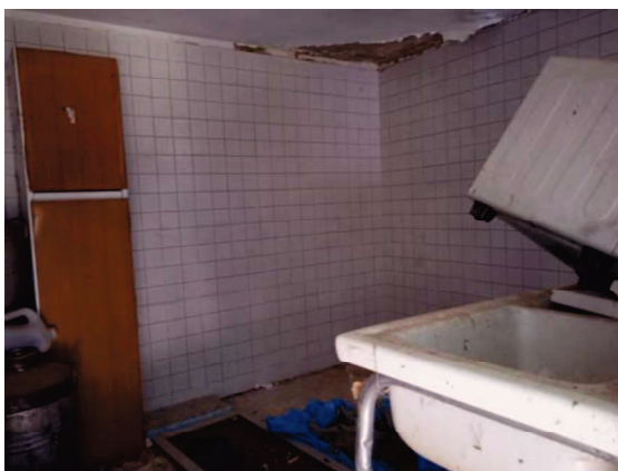
Part. 405 sub 5 - Vista interna piano seminterrato
