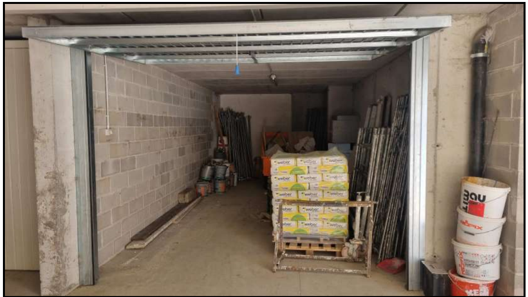
GARAGE Piano interrato
