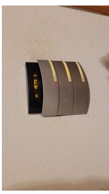
L7_Villa unifam._01 piano seminterrato (9)
