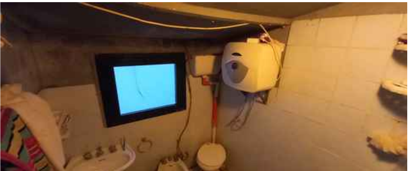
Piano Terra – BAGNO
