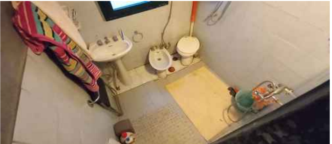
Piano Terra – BAGNO
