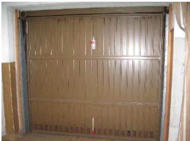
Locale accessorio exautorimessa (PS1)
