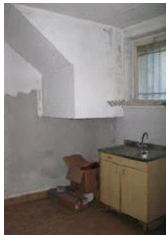
Locale accessorio exautorimessa (PS1)
