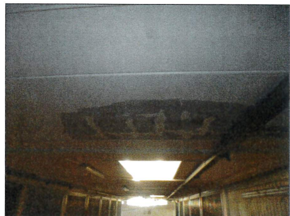
Vista piano interrato
