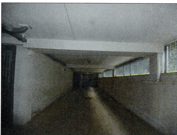
Vista piano interrato
