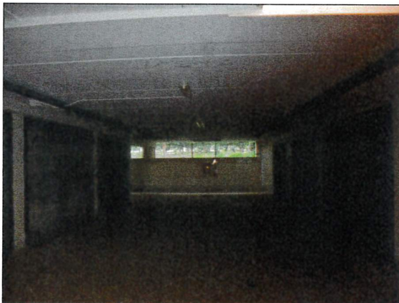
Vista piano interrato
