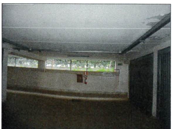
Vista piano interrato
