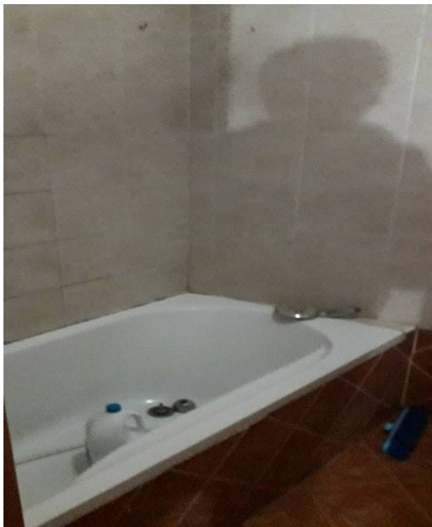
Bagno piano terra
