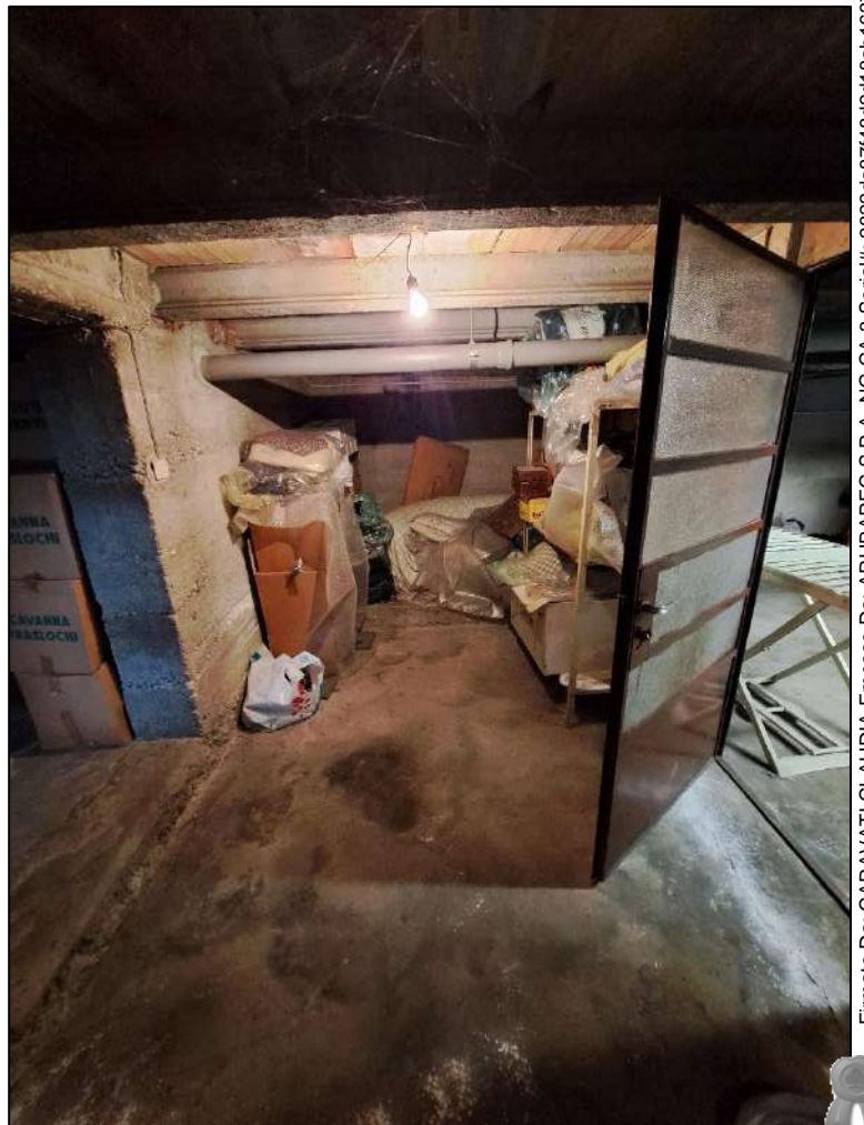
Piano seminterrato Intercapedine (cantina)
