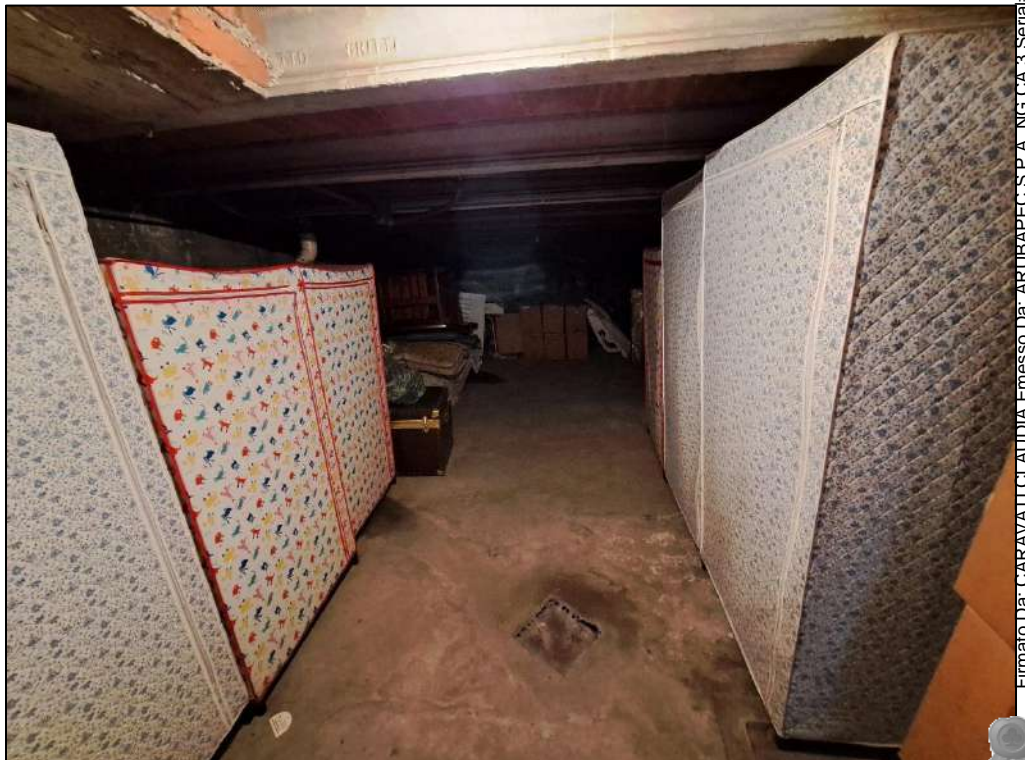
Piano seminterrato Intercapedine (cantina)
