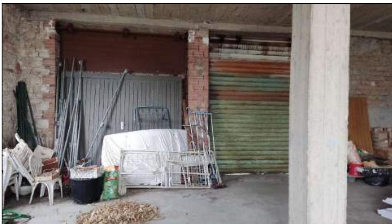
vista garage piano terra
