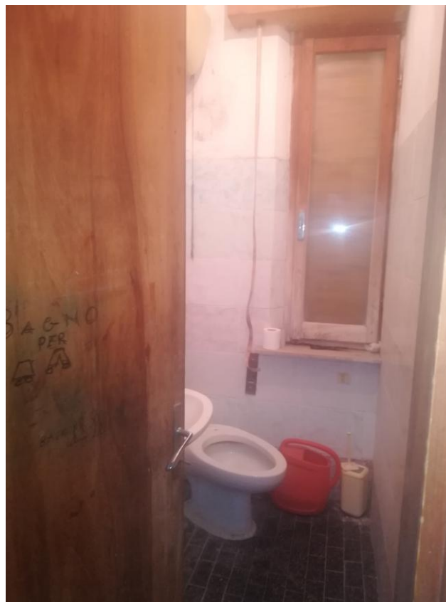
SUB. 24-PIANO TERRA : INTERNO WC
