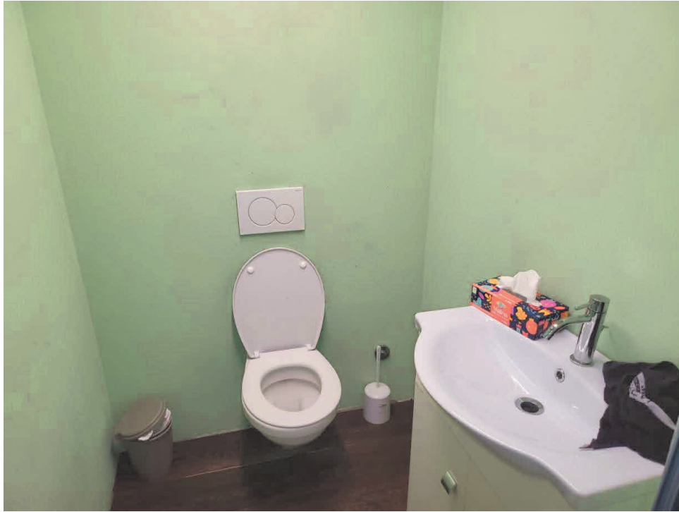
Piano terra Bagno (foto 17/07/2023)
