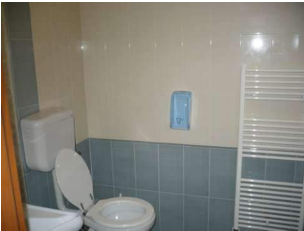
Bagno – piano terra
