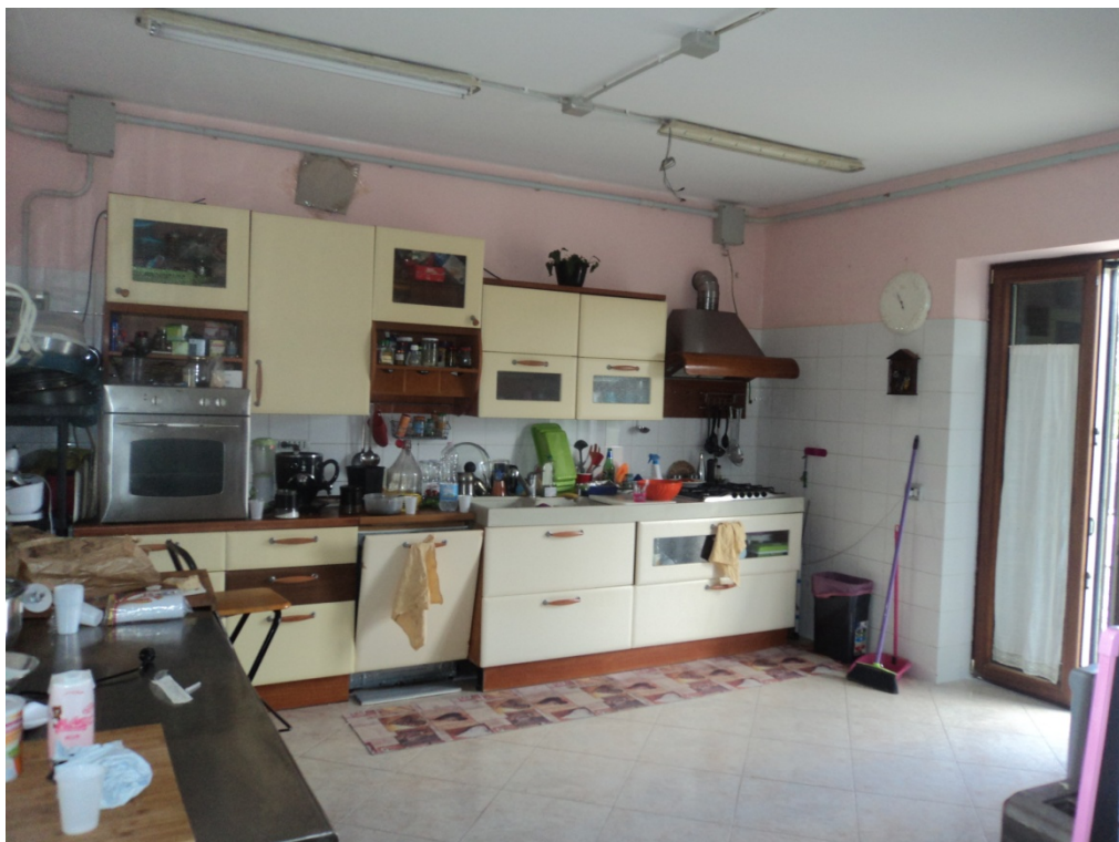
PIANO TERRA – Locale adibito a “country house”
