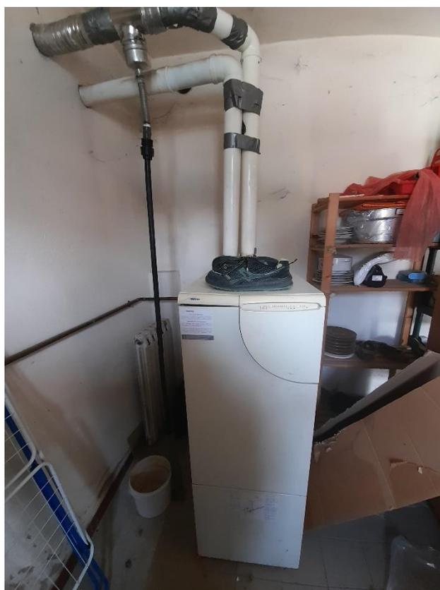
FOTO 17 – Caldaia a gas
