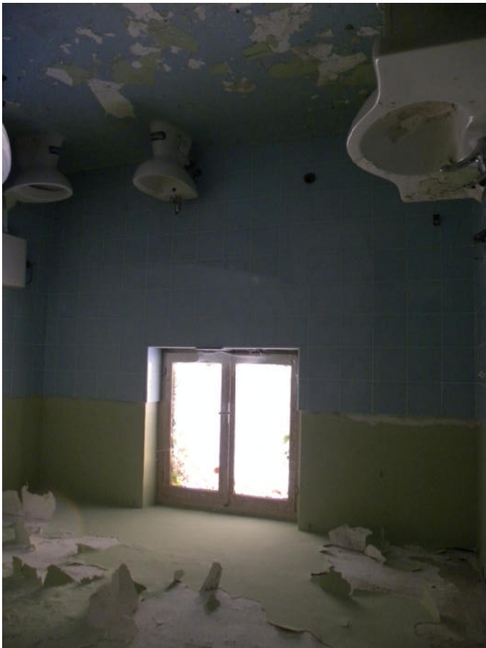
BAGNO PIANO TERRA
