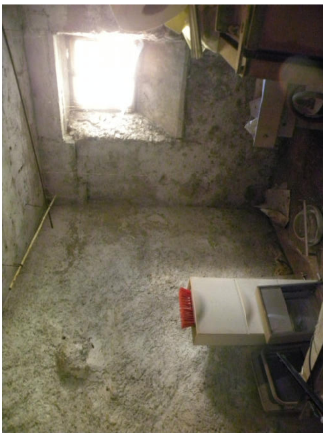
CANTINA PIANO TERRA
